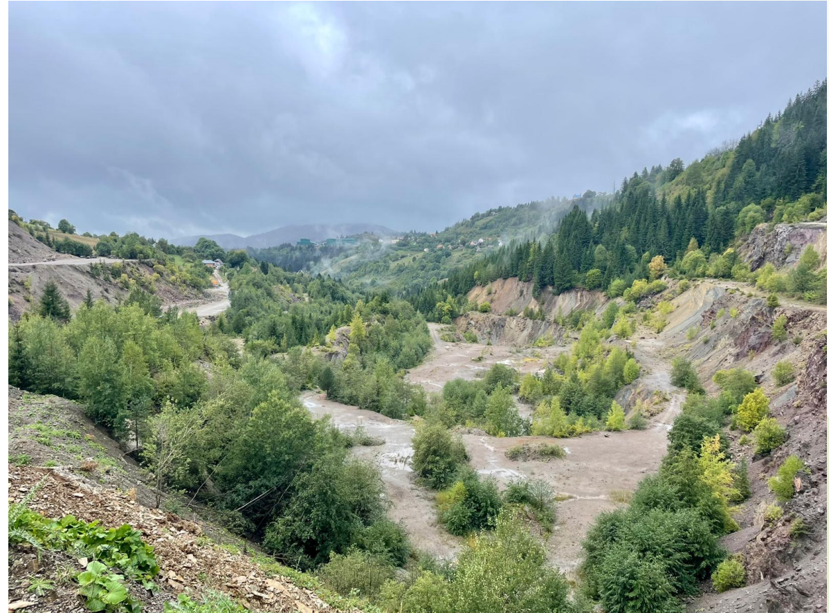
Veovaca Tailings Storage Facility
